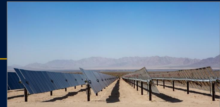
Oberon Solar and Storage Facility Riverside County, CA
